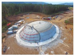
Figure 1: Inflated dome - pilot construction realized in 2017 by ÖBB, the Austrian rail operator as a wildlife crossing over railroad tracks
